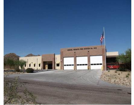
STATION 403 5960 S. Cardinal Ave Built 1974 Replaced 2009 Battalion 415 Engine 423 Ambulance 433 Squad 443
