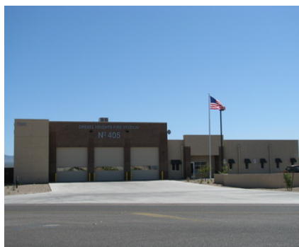
STATION 405 7200 S. Wade Road Built 2010 Engine 425
